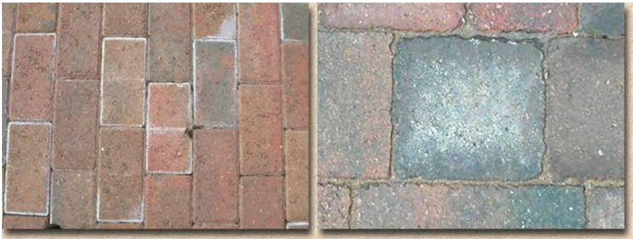
Efflorescence that appears only at the edges, or in distinct central bands, as seen in this image, probably results from poor storage after manufacture and curing
