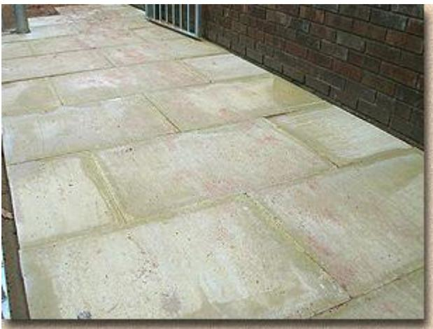
BS flags can be prone to efflorescence because of their relatively high cement content
