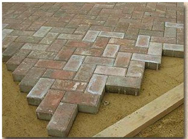
Bloom evident on brand new paving is most likely to be primary efflorescence
