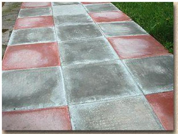
Paving that has been down for some time is more likely to suffer from secondary efflorescence
